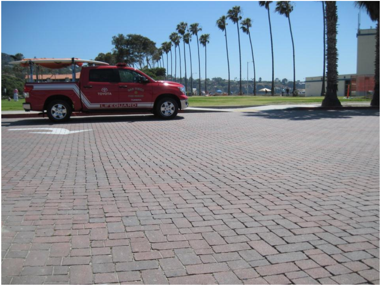
Figure A.3-1. Permeable interlocking concrete pavement.
